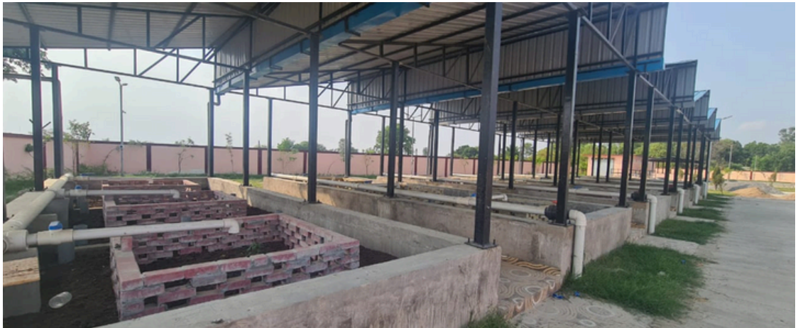
Image 9: 32 KLD capacity Faecal Sludge Treatment Plant (FSTP)
