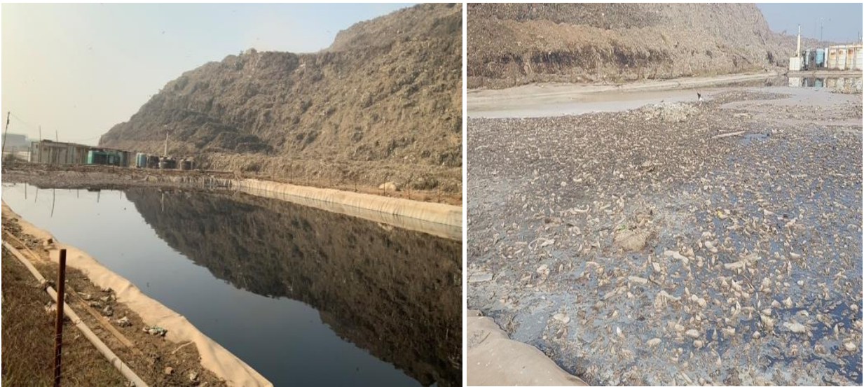
Fig. 5: Onsite leachate Collection Pond
