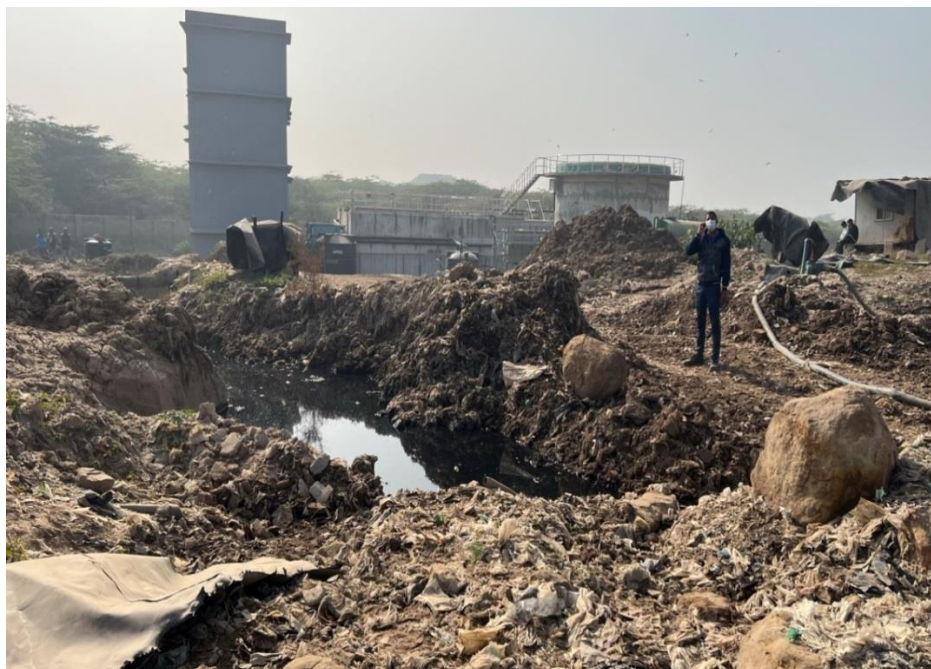
Fig. 4: Improper drainage system for leachate collection
