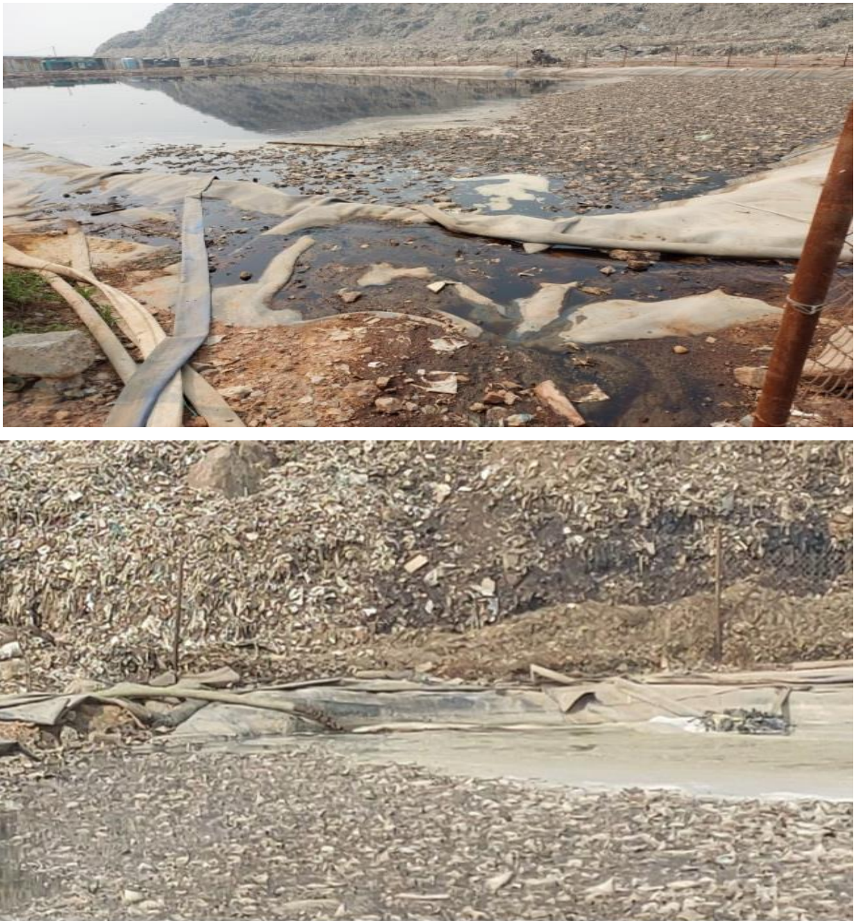
Fig. 9: Improper maintenance of leachate storage system at DTRO unit
