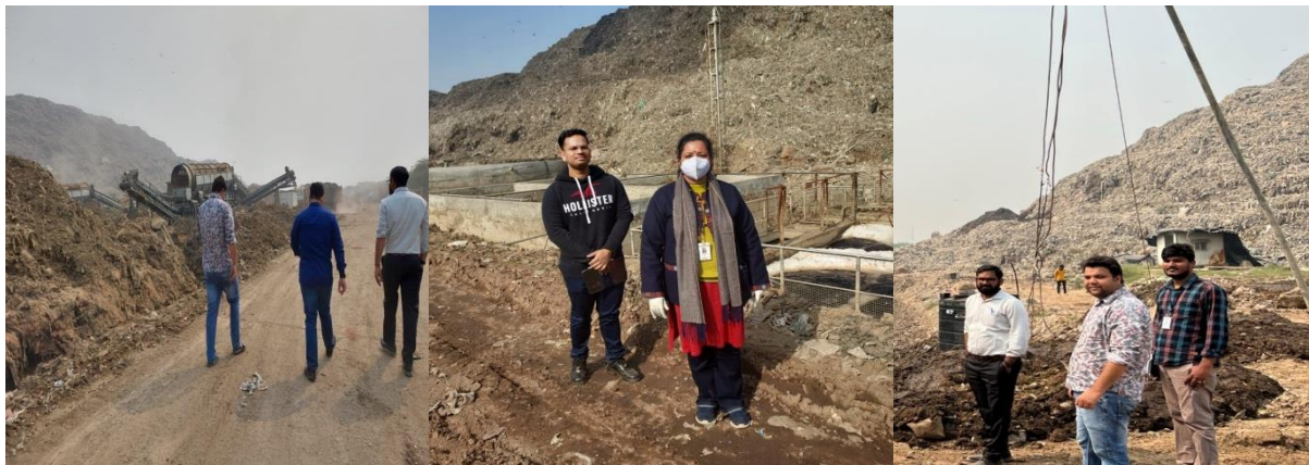
Fig. 2: Entrance way to reach landfill site and different leachate treatment units
