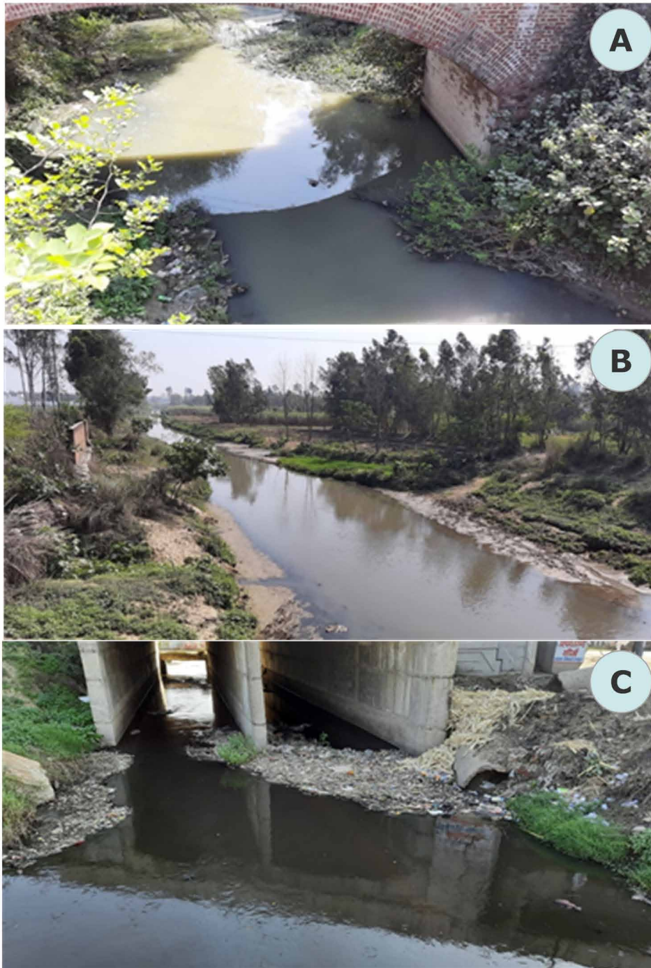
Figure 4. (a) Pachhana drain; (b) Dhandi drain; and (c) Rampur drain
