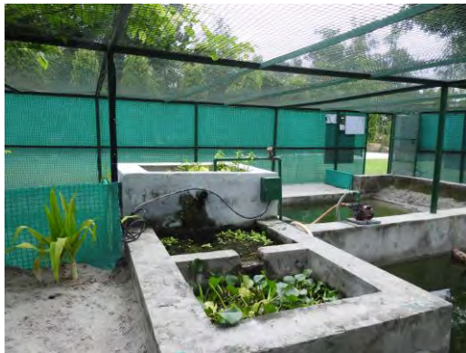
Fig: Bio-filtration Unit of Enclosure I
