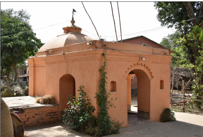
Figure 36: Mahavir Mandir, Shahpur Source: Primary survey by AH Division, INTACH.
