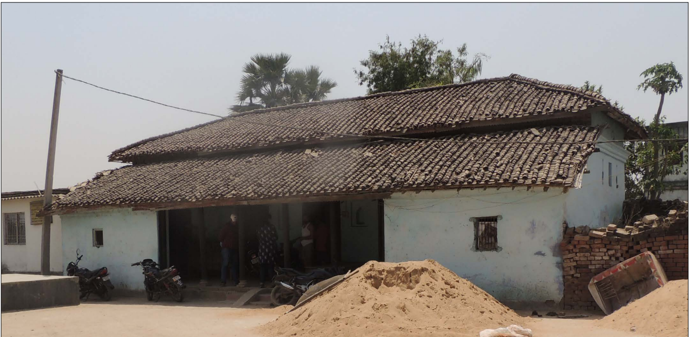
Figure 32: Vernacular residence in Bhojpur tehsil
