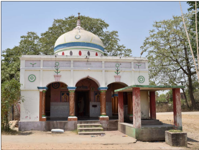
Figure 29: Shiv Temple, Suhiya, Bhojpur district Source: Primary survey by team, AH Division, INTACH
