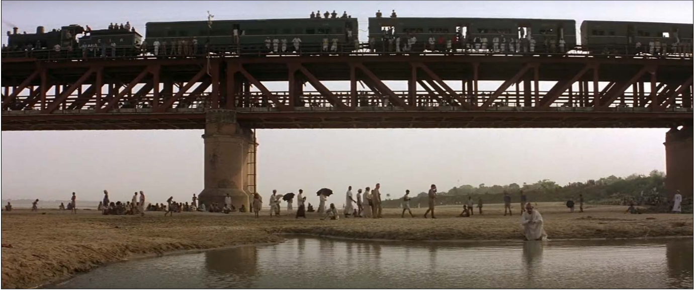
Figure 9: Koilwar bridge, featured in 1982 film, Gandhi
