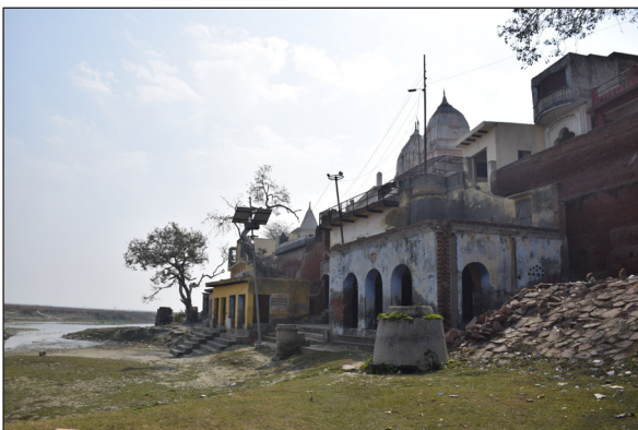
Figure 4: Mansoori ghat, Anupshahr Source: Primary survey, site visited on 3rd February, 2021
