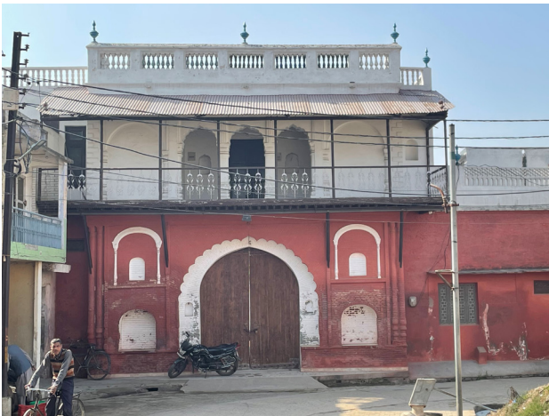
Figure 22: A Residence in Bugrasi, Siana tehsil Source: Primary survey by team, AH Division, INTACH
