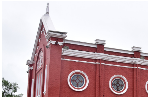
Figure 54 Ornamental pediments and tracery moulding in churches (Source - Primary survey, visited on 18 th August, 2019.)
