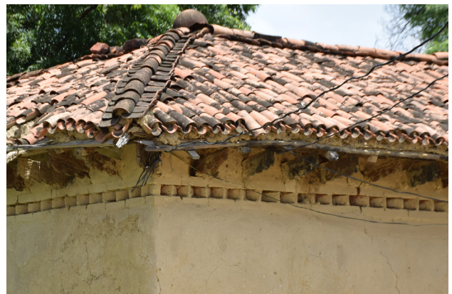
Figure 43 Small openings and brackets use in mud houses. (Source - Primary survey, visited on 17 th August, 2019.)
