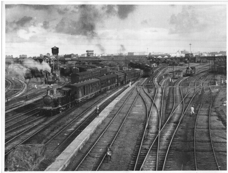
Figure 30 The Mughalsarai railway station at Chandauli.
