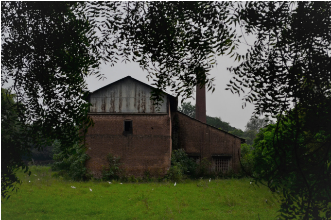
Figure 35 : Glass Factory in Najibabad tehsil. Source: Primary study by AH Division, INTACH Team
