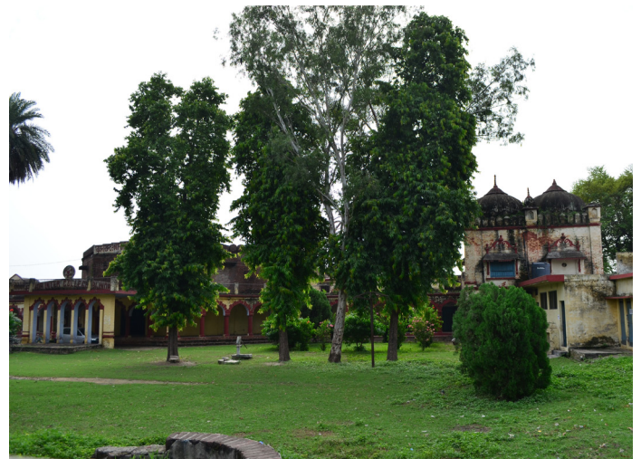
Figure 23: Bijnor Inter College, Bijnor Source: Primary study by AH Division, INTACH Team
