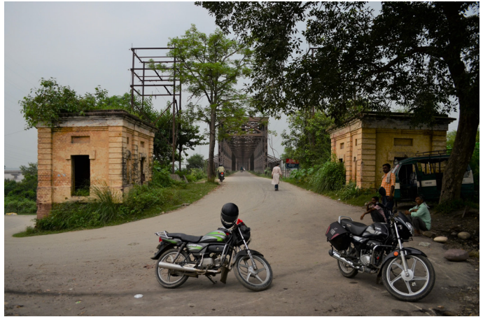
Figure 36 : Railway bridge over Ganga in Balawali village. Source: Primary study by AH Division, INTACH Team
