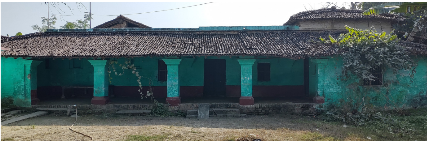
Figure 4: Lakshman Shah’s Residence, Mohanpur tehsil Source: Primary survey by AH Division, INTACH Team
