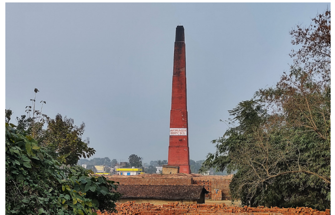
Figure 49: Brick Kiln, Vidyapati Nagar Source : Primary Survey by AH Division, INTACH Team
