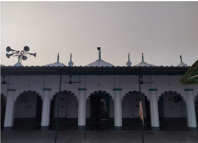
Figure 23: Jama Masjid at Mohiuddinnagar Source: Primary survey by AH Division, INTACH Team
