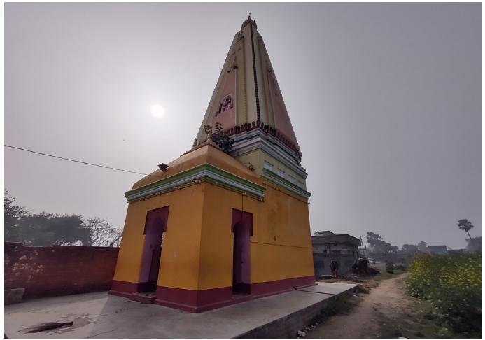
Figure 21: Shiv Mandir at Vidyapati Nagar Source: Primary survey by AH Division, INTACH Team
