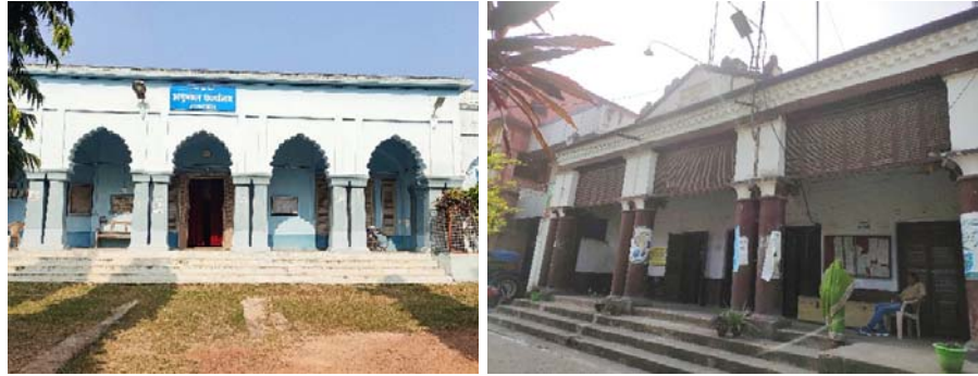
Figure 33 a) Palace remains reused as the Anumandal Karyalaya b) Nagar Parishad Sahibganj. Source: Primary site visit
