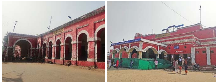
Figure 47 Railway stations at a) Rajmahal and b) Sahibganj. Source: Primary site visit.
