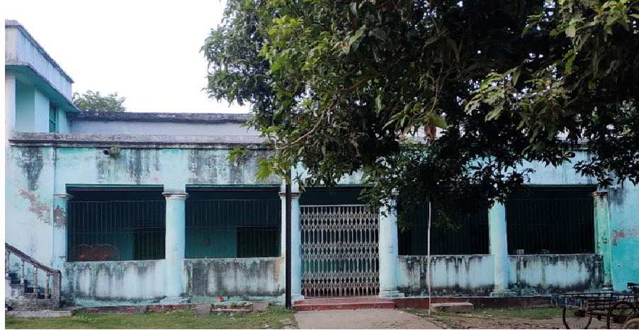
Figure 48 Neel Kothi, Rajmahal. Source: Primary site visit.
