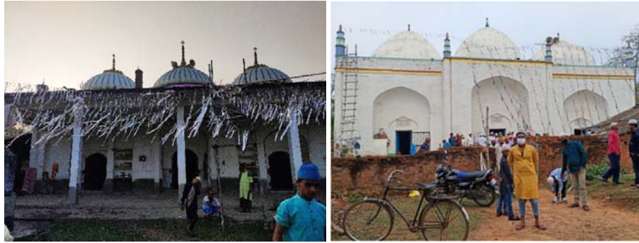
Figure 30 a) Nayabasti Masjid b) Roshan Masjid. Source: Primary site visit.
