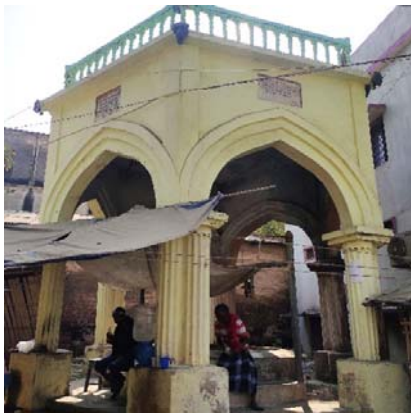
Figure 40 Bhagwan Kuan. Source: Primary site visit.
