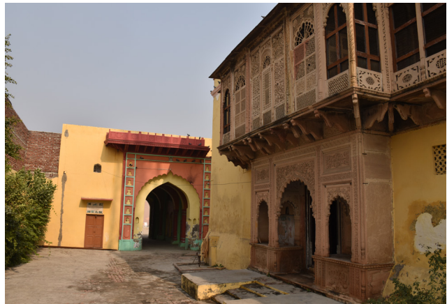
Figure 24: Internal courtyard of Pratap Singh ki Garhi, Gawan Source: As per primary survey done on site
