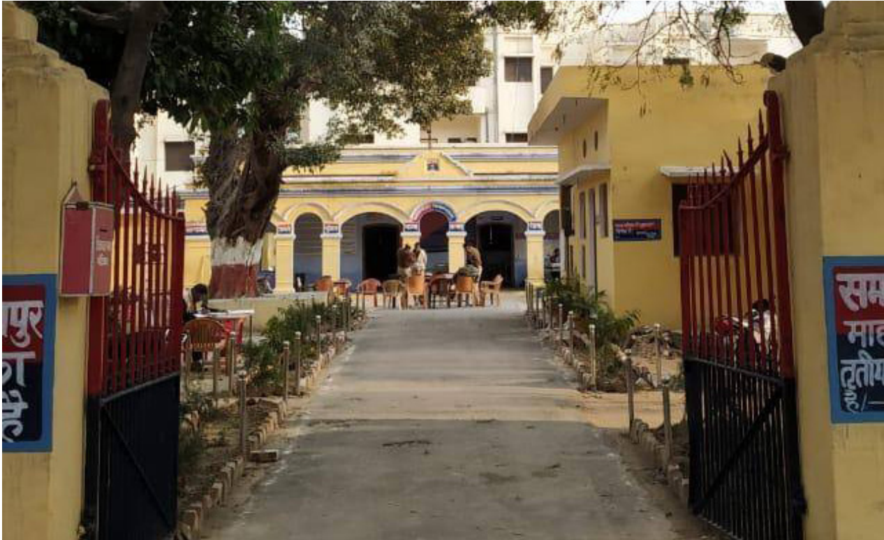
Figure 8: Alapur police station, Dataganj tehsil
