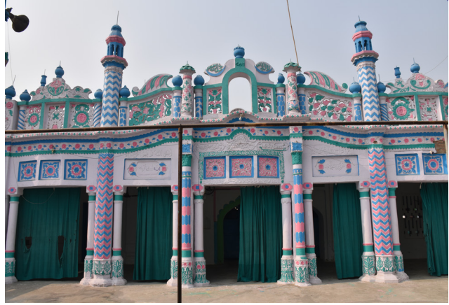
Figure 22: Arcaded corridor of the Jama Masjid, Nadail Source: As per primary survey done on site
