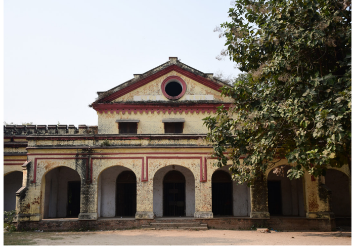
Figure 29 : GIC High School, Ballia City Source: Primary study by AH Division, INTACH Team
