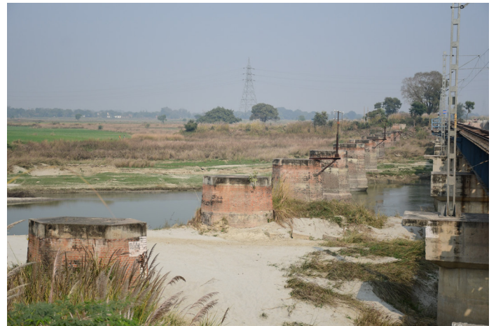
Figure 26 : Tamsa River Bridge Source: Primary study by AH Division, INTACH Team
