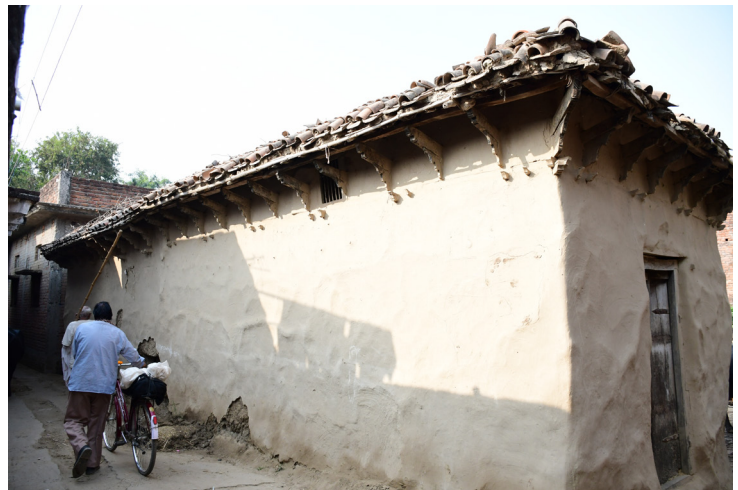
Figure 16 : Mud house in Shrawanpur
