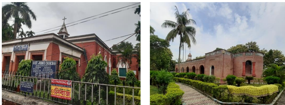
Figure 33 St. John's Church, Berhampore and b) Armenian Church, Berhampore. Source: Primary survey by Mr. Balaknath Bhattacharya.
