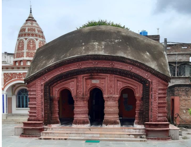
Figure 26 Jor Bangla roof of Dayamoyee Kali Mandir. Source: Primary Visit by Mr. Balaknath Bhattacharyya
