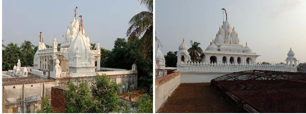
Figure 34 a) Shri Neminathji Temple and b) Shri Chintamani Parasnath Temple at Azimganj. Source: Primary Survey by Mr. Balaknath Bhattacharyya
