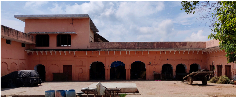
Figure 31: Imambara, Kakrauli, Muzaffarnagar Source: Primary study by AH Division, INTACH Team
