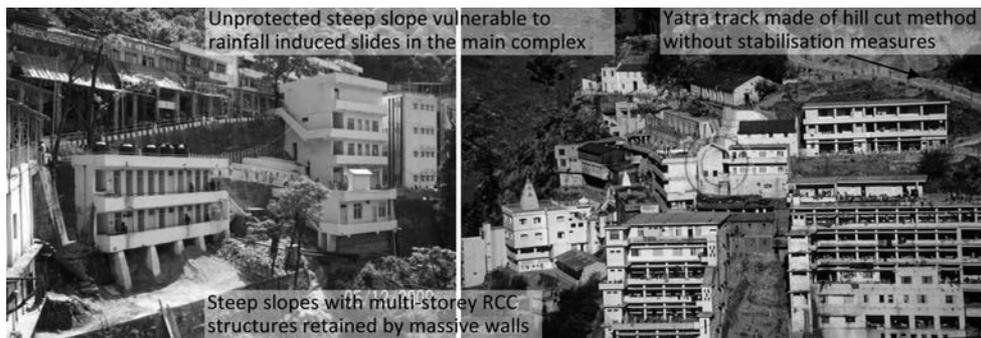
Figure 8: Vulnerable multi-tier infrastructures in the main Bhavan complex leaving little or no scope for effective rescue operations during earthquake and rainfall induced land slippages.
