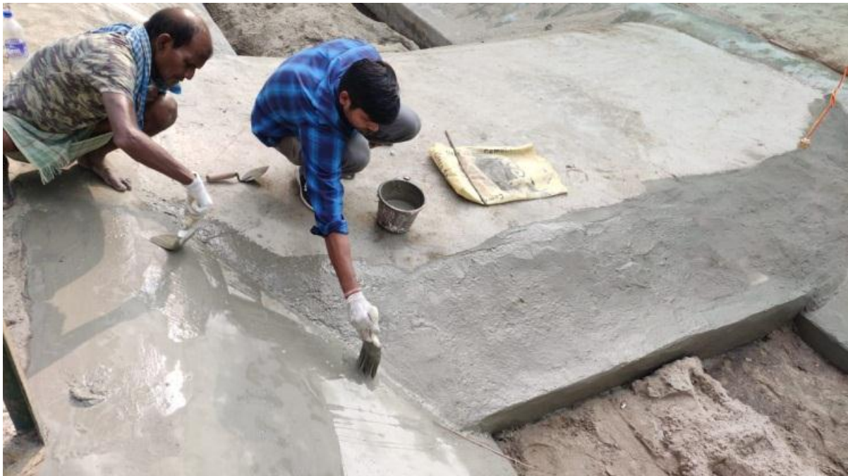
Application of a coating of waterproofing mixture
