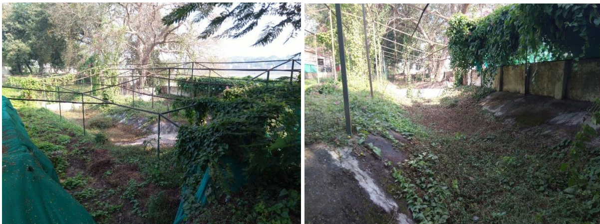
State of enclosure III before beginning refurbishment work
