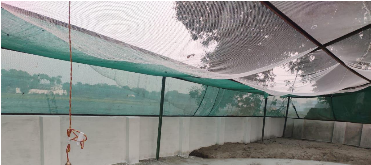
Covering the top of the enclosure
