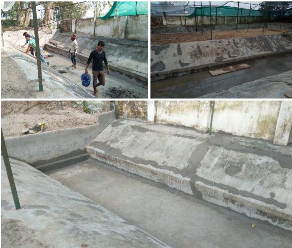
Sealing cracks in the water-body
