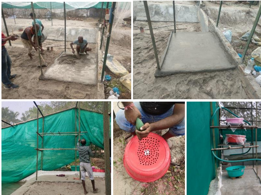
Setting up the filtration unit
