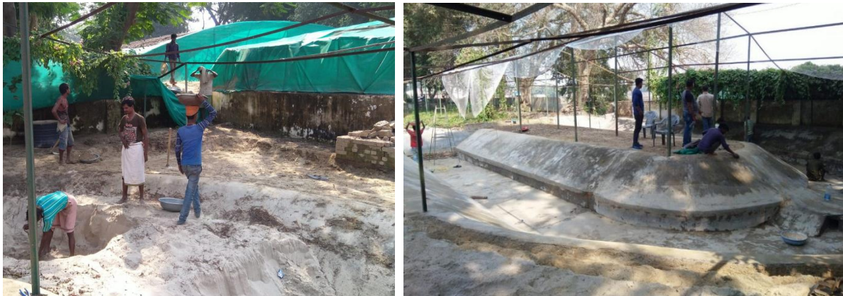
Enclosure III being cleared of sand
