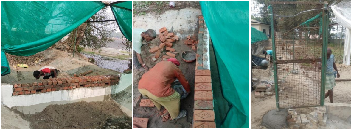
Reinforcing the enclosure partition and installation of gate
