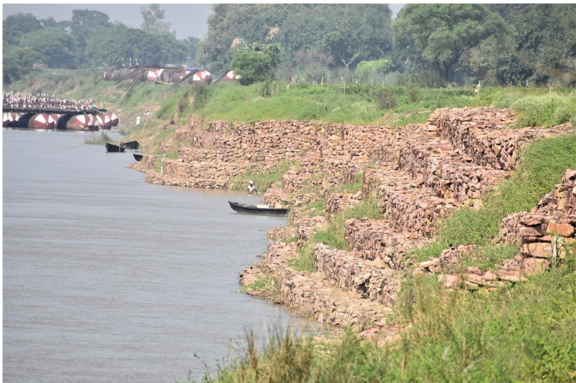
Image 44 : Erosion Control With Gabions Along Ganga Bank Near Narainpur
