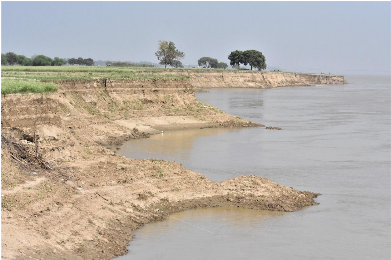
Image 42 : Ganga River Bank Erosion As Observed Near Hathikhana Village In Ghazipur
