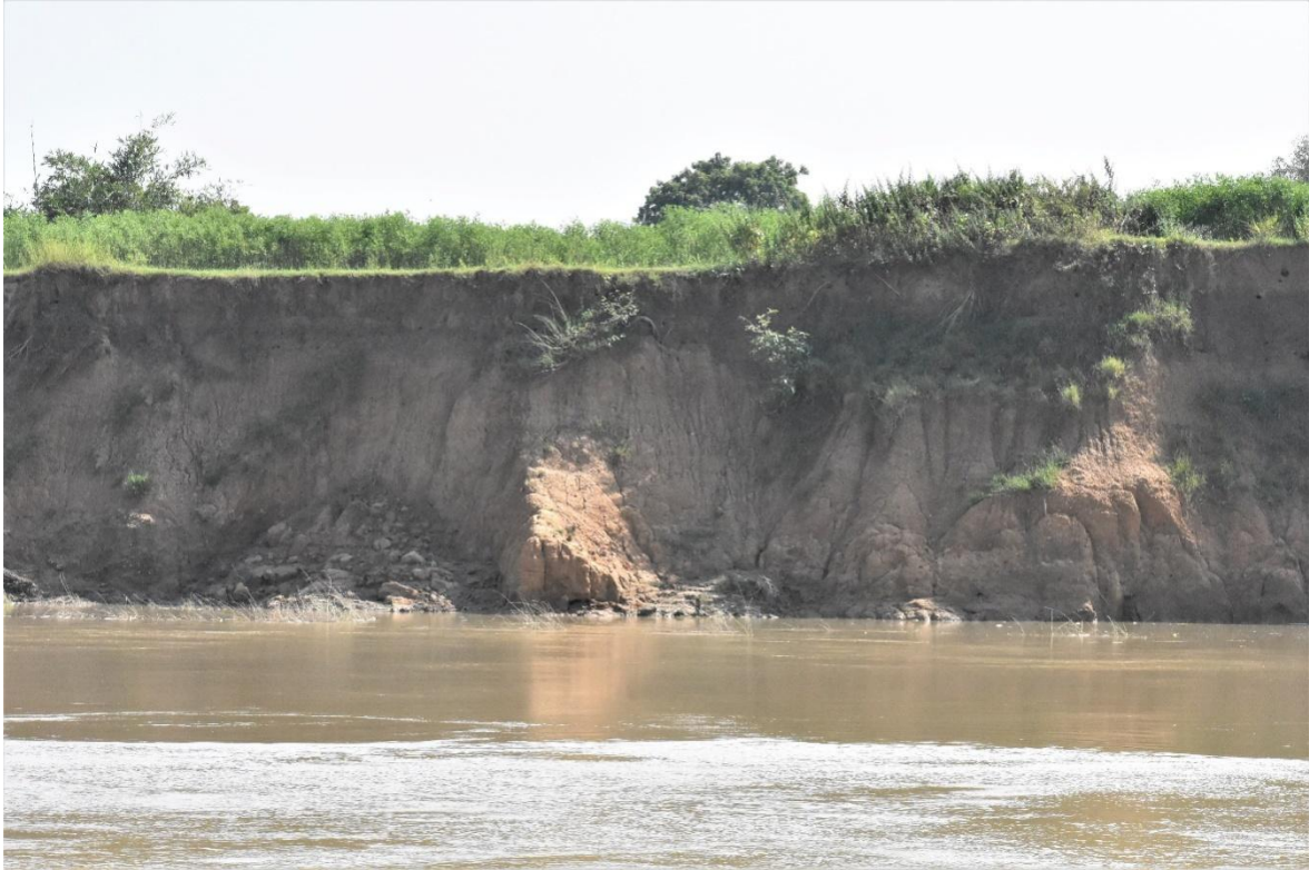
Image 43 : Ganga River Bank Erosion As Observed Near Gahmar Village In Ghazipur
