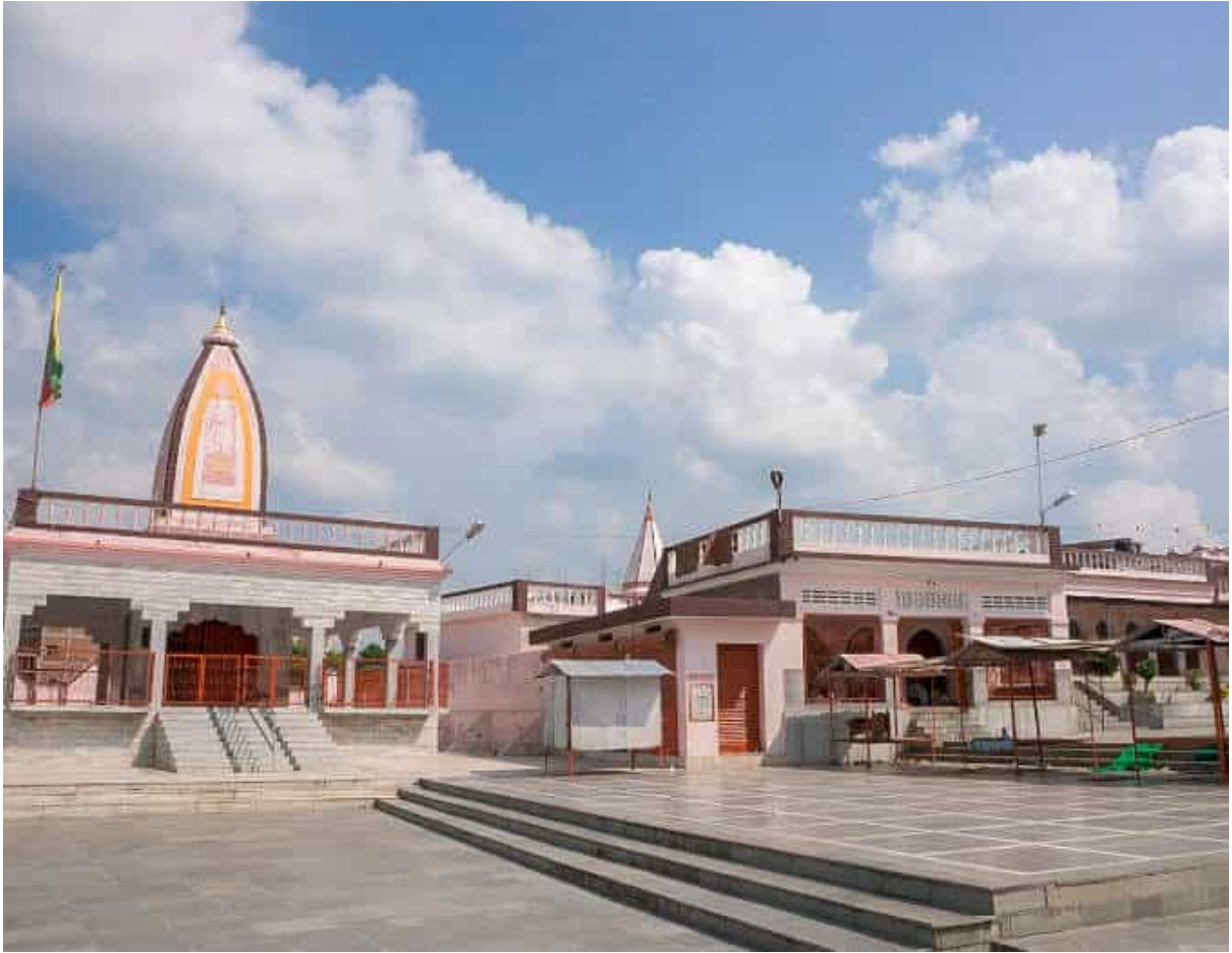
Figure 25A view of Bela Bhawani Temple Source https://www.justdial.com/photos/belha-devi-pratapgarh-uttar-pradesh-temples-lyjwikfmt7-pc-107259173-sco-99iimyeyui
