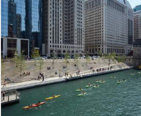
Trees are integrated into the staircase with a custom design.
