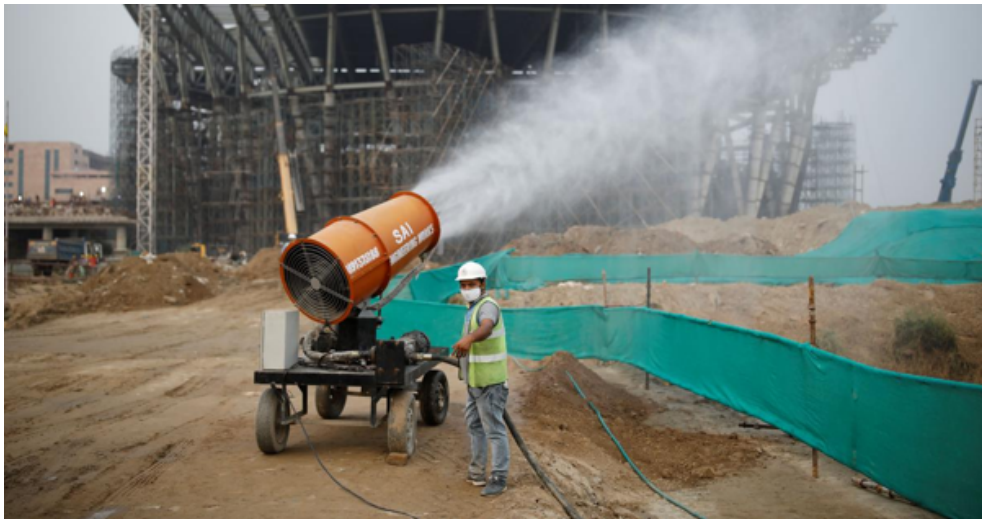
A worker operates an anti-smog gun at a construction site in New Delhi Source: Adnan Abidi/ Hindustan Times (2022)
