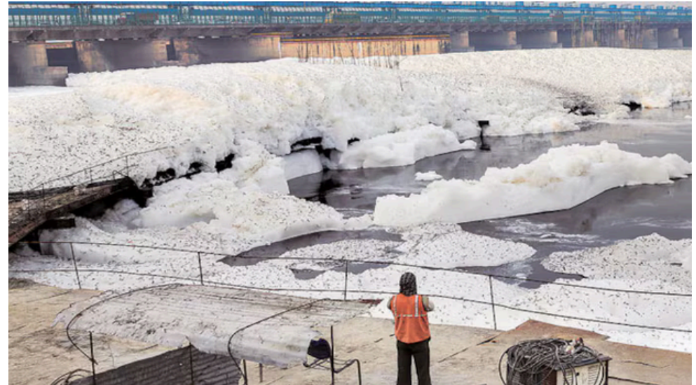
Industrial discharge flows directly into the Yamuna through rainwater drains
