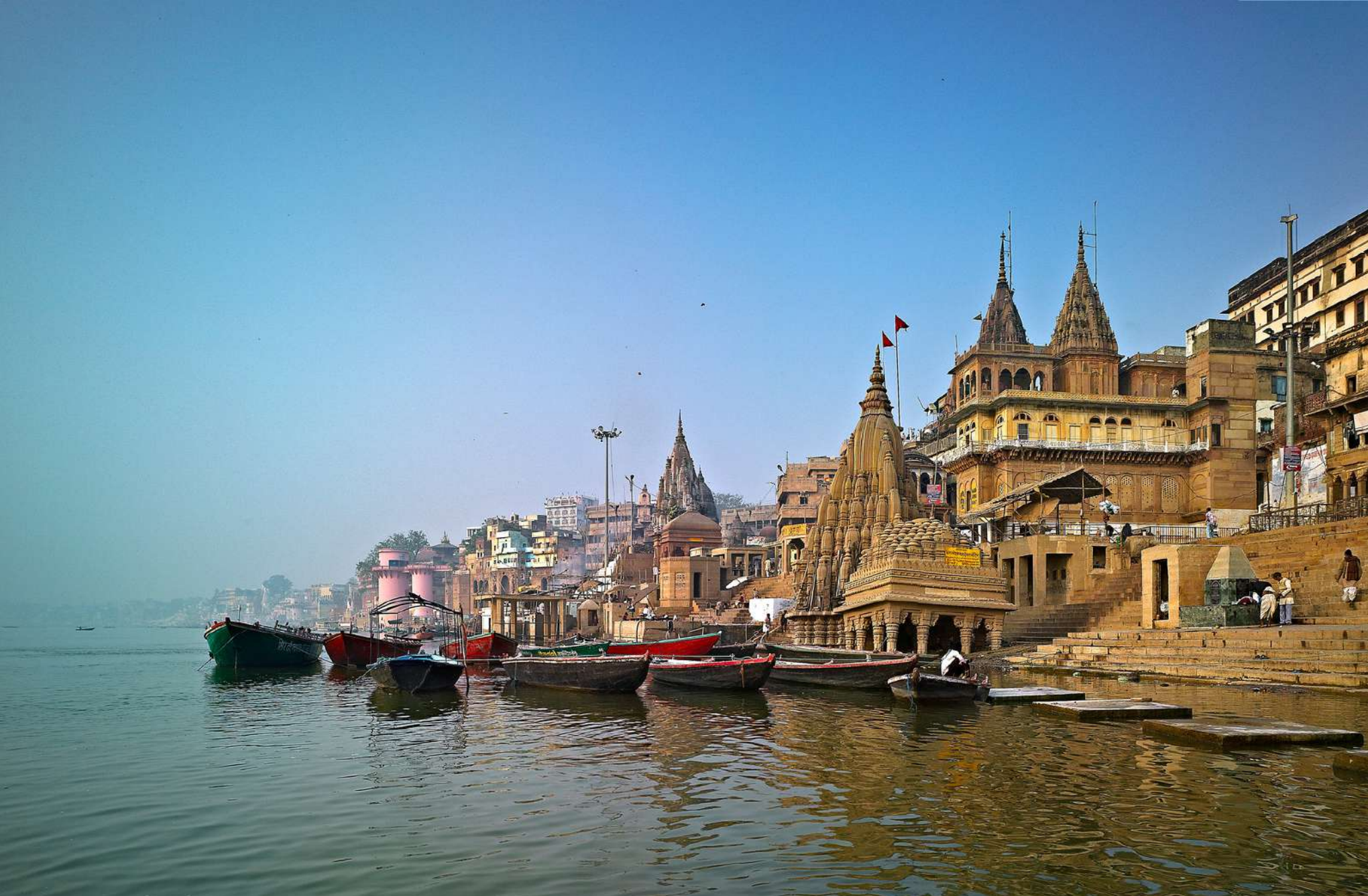
Improvement of 26 Ghats along the Ganga River stretch
