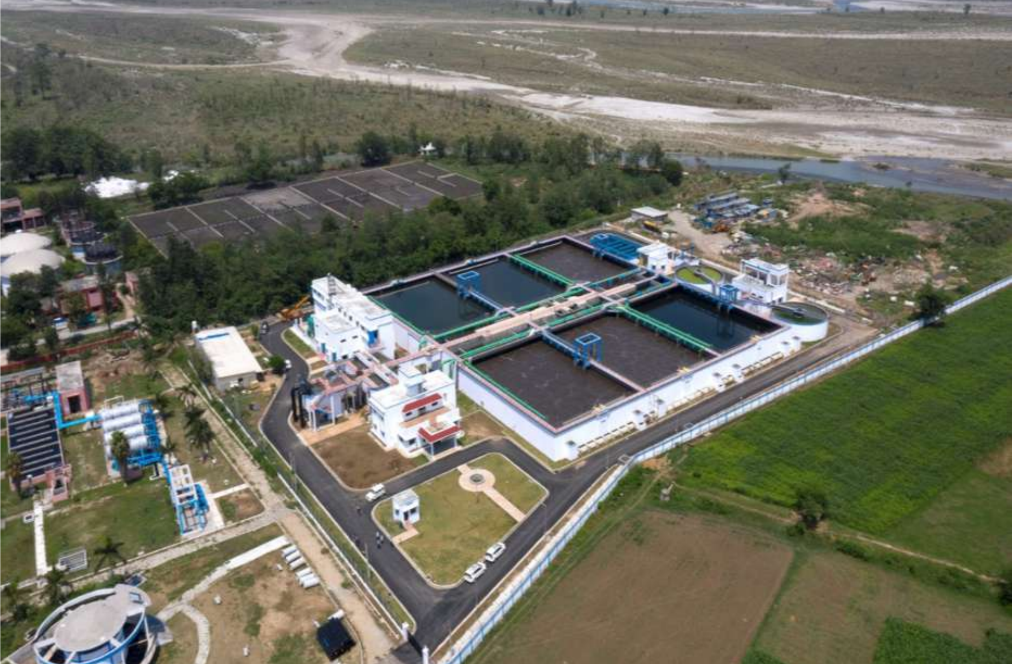
Glimpse of 68 MLD STP in Haridwar (Source - NMCG)
