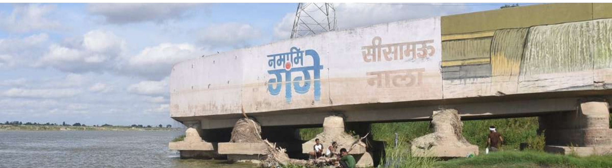
The infamous 140 MLD Sisamu Nala before and after the tapping (Source - NMCG)
