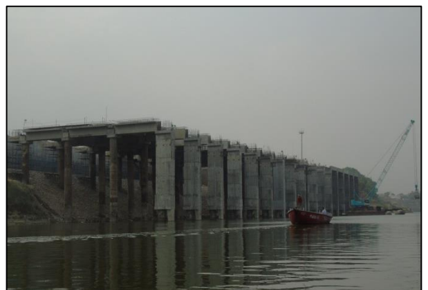
Construction of Jetty near Ramnagar
