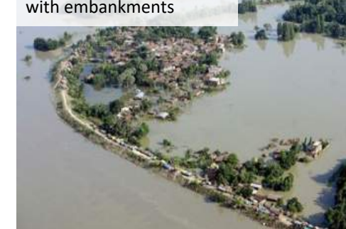
Cleaner river, protected with embankments
