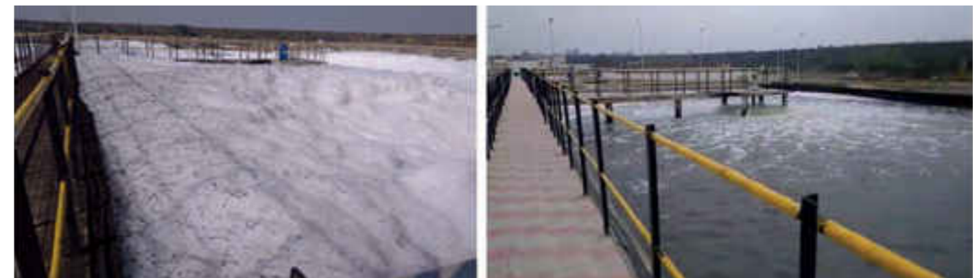
BIO-REMEDIATION OF 60 MLD STP AT RAJAPUR, ALLAHABAD (RECEIVING 95 TO 100 MLD SEWAGE), UTTAR PRADESH, INDIA
