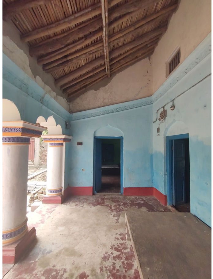
Figure 33: Verandah of Manohar Singh's Residence showing the roofing system. Logs are used to support the sloping roof, Mahnar Source: Primary survey by AH Division, INTACH Team
